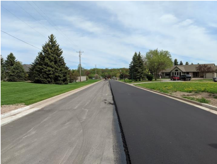
Completed East Side Pavement Looking North From Prairie Song Lane
