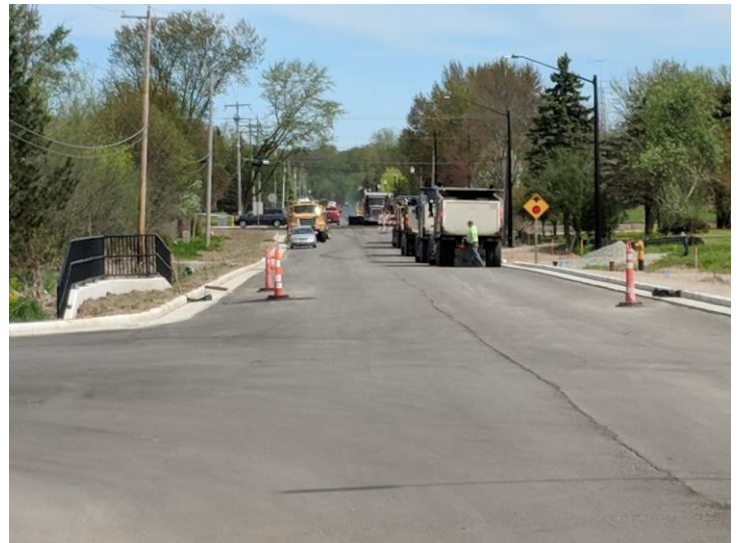
Paving Operation Looking North Towards Capitol Drive
