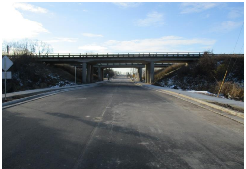
Looking south under I-41
