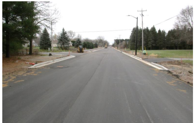
Constructing Curb Ramps at Elsner Road
