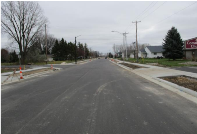
Completed Asphalt Lower Layer and Sidewalk
