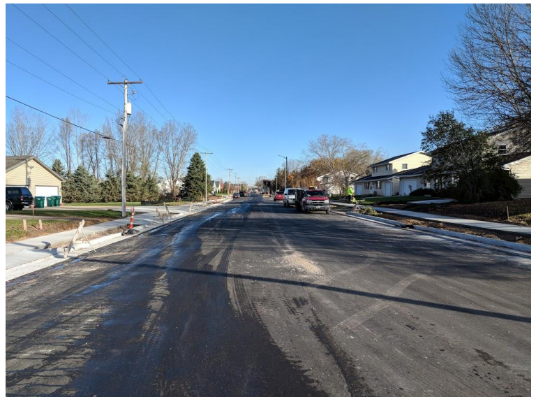
Completed Lower Layer Pavement
