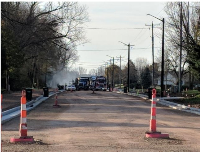
Paving Lower Layer Asphalt
