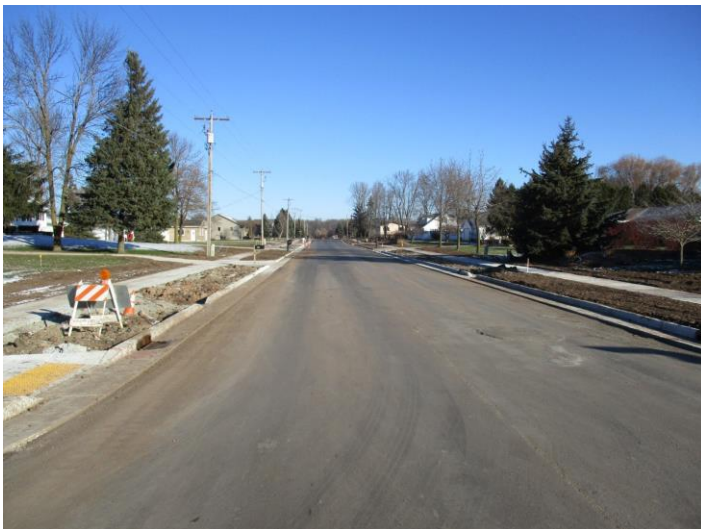
Looking North from Amberwood Lane
