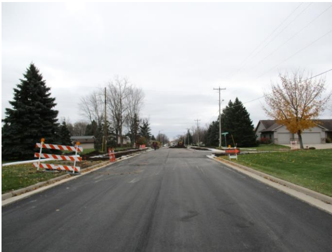
Backfilling Terraces South of Prairie Song Lane
