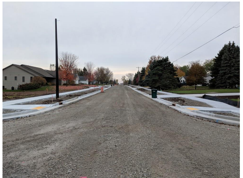
Street Prepped for Lower Layer Asphalt
