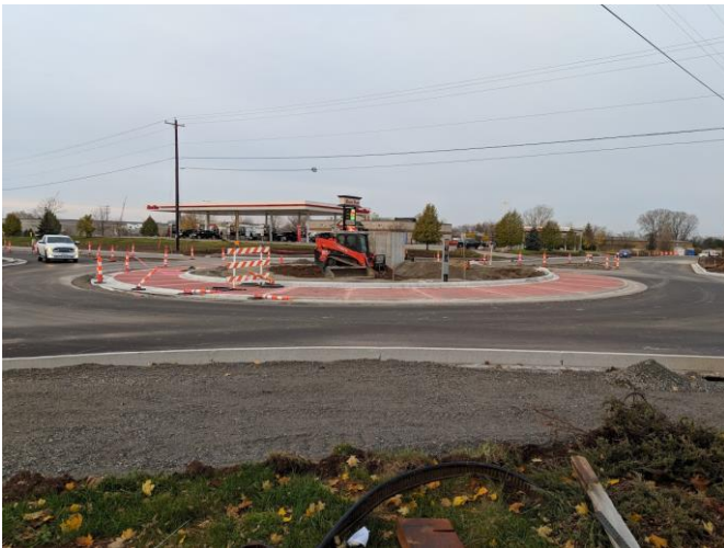
Grading Victory Lane Roundabout Center Island
