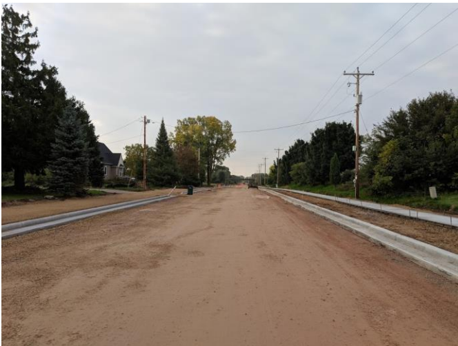
Completed Curb & Gutter and Sidewalk
