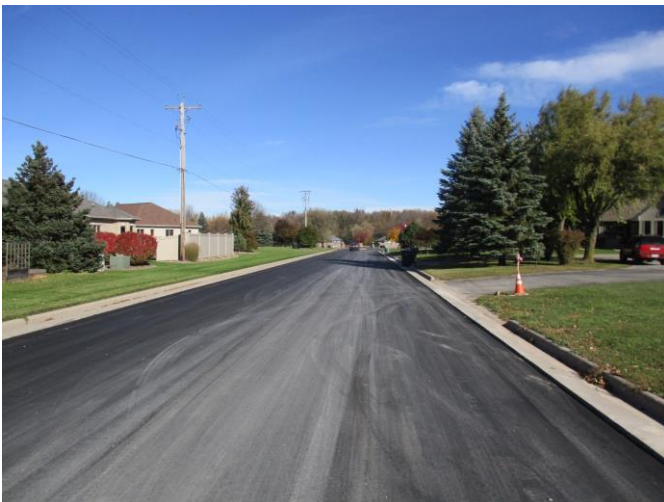
Asphalt Lower Layer Placed North of Prairie Song Lane
