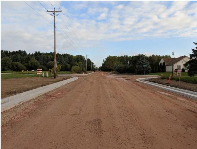
Completed Street Base and Curb & Gutter Looking North From Starview Drive
