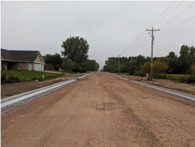
New curb and gutter placed on N. Gillett Street
