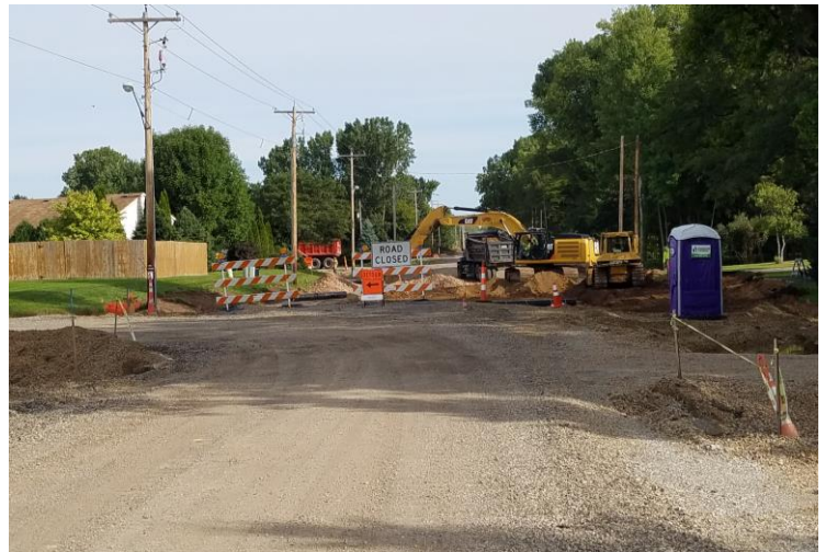
RC Excavating placing road base between Rachel Lane and Kaylee La
