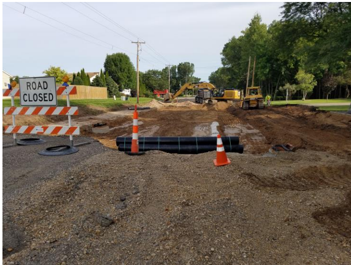
RC Excavating digging down to subgrade
