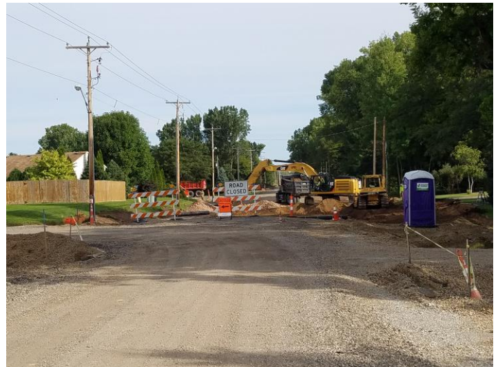
RC Excavating placing road base between Rachel Lane and Kaylee Lane
