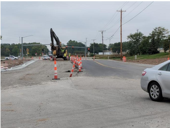
Placing Base Course in Victory Lane Roundabout
