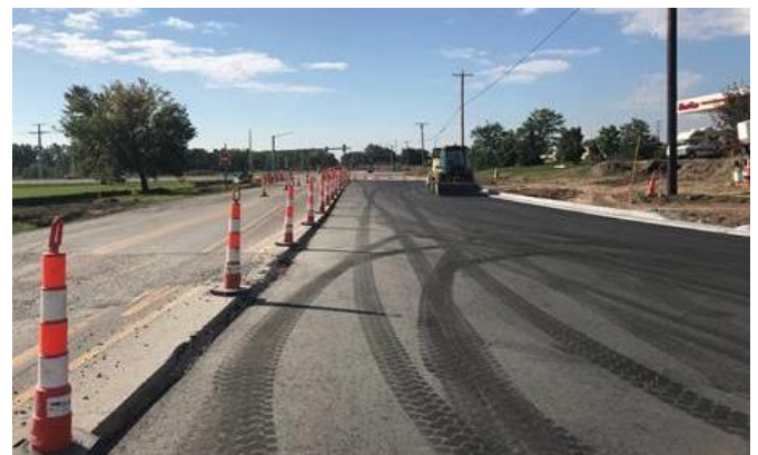
Looking south from Victory Lane at lower layer of asphalt/curb & gutter
