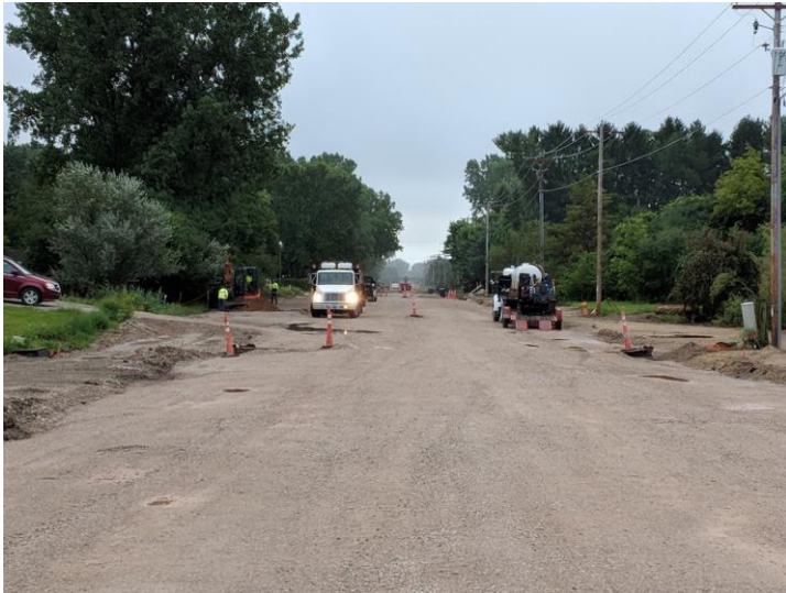
Relocating Cable TV South of Starview Drive
