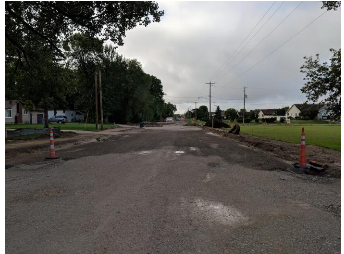
Roadway Grading and Graveling North of Little Ranch Road
