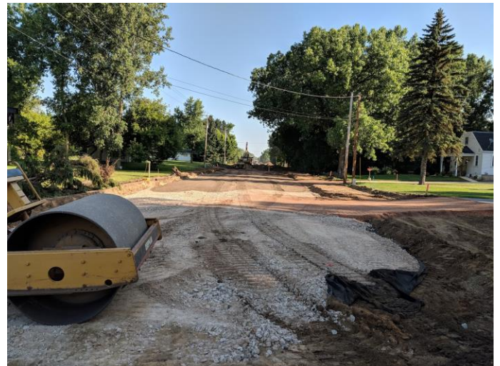
Placing Aggregate Base Course Looking North From Little Ranch Road
