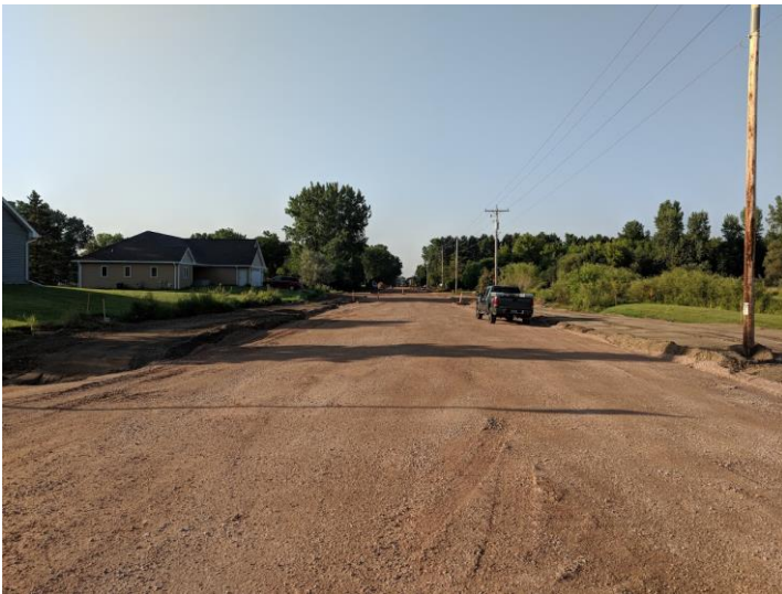
Completed Base Course Looking South From Starview Drive
