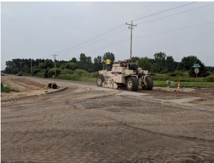
Milling Off Asphalt Pavement
