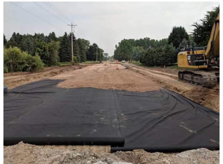
Excavating Street and Placing Aggregate Base
