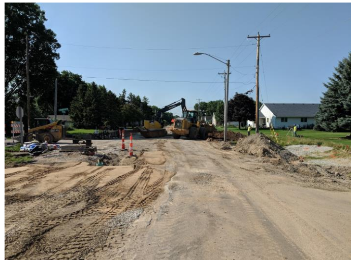
Storm Lateral Installation at Hiawatha Drive
