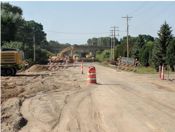
Storm Lateral Installation North of I-41
