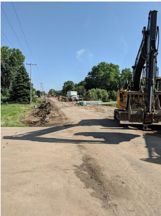
Installing Storm Sewer North of Capitol Drive
