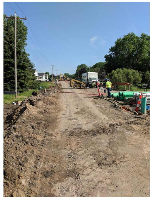
Installing Storm Sewer at Creek Crossing
