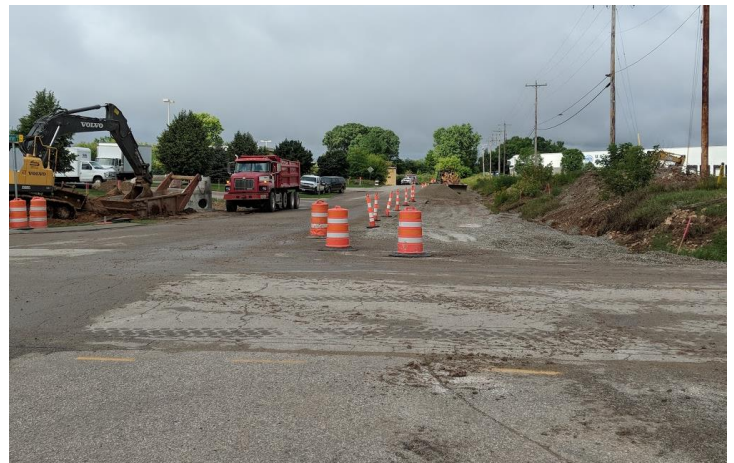
Constructing Temporary Widening on Victory Lane
