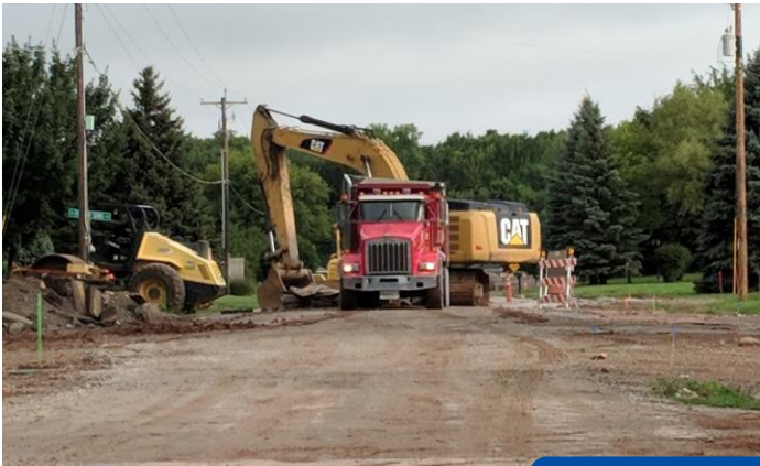
Excavating and Placing Aggregate Base at Prairie Song Lane
