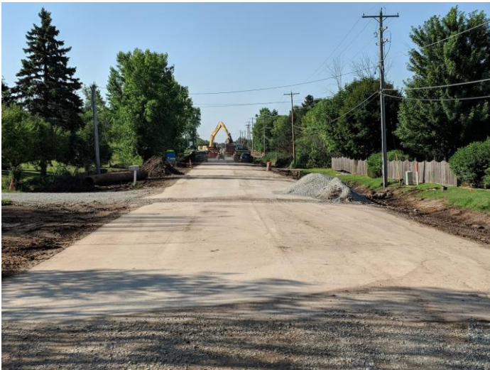
Installing Storm Sewer South of Capitol Drive
