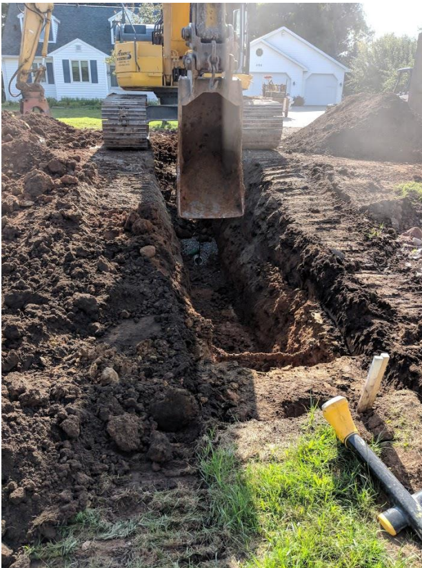
Installing Storm Lateral
