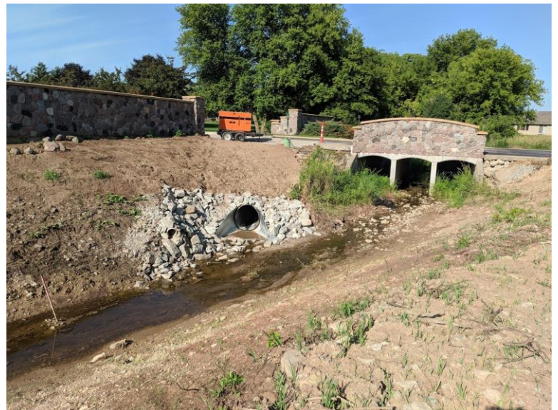
Storm Sewer Outlet to Grand Chute - Center Drain
