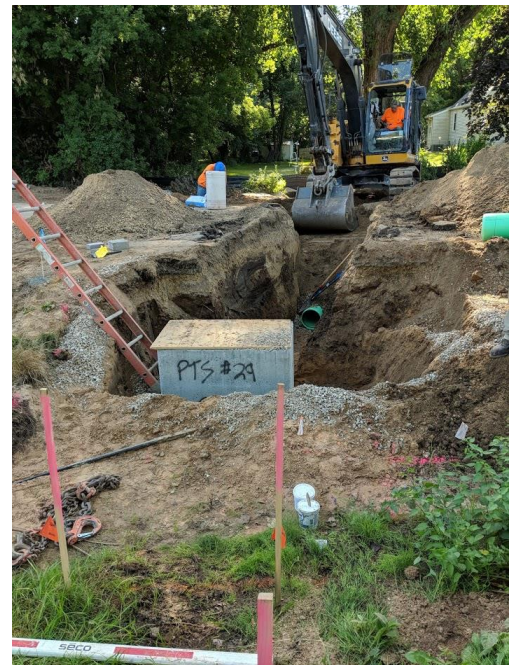
Installing Inlet Lead North of Little Ranch Road
