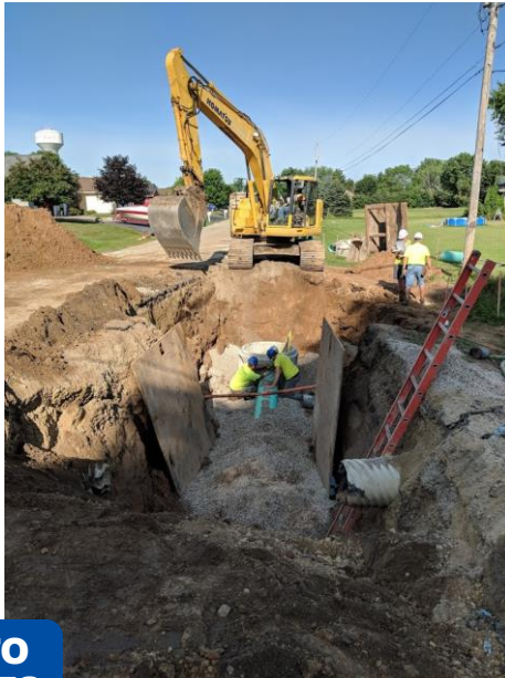
Installing Storm Sewer at Little Ranch Road
