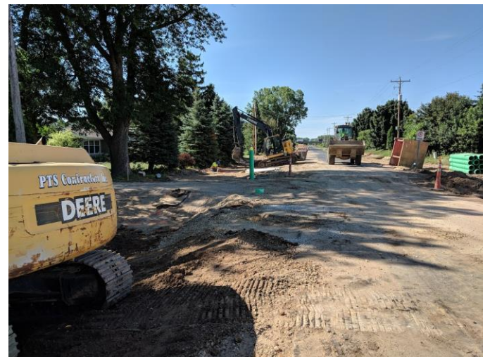
Installing Storm Lateral
