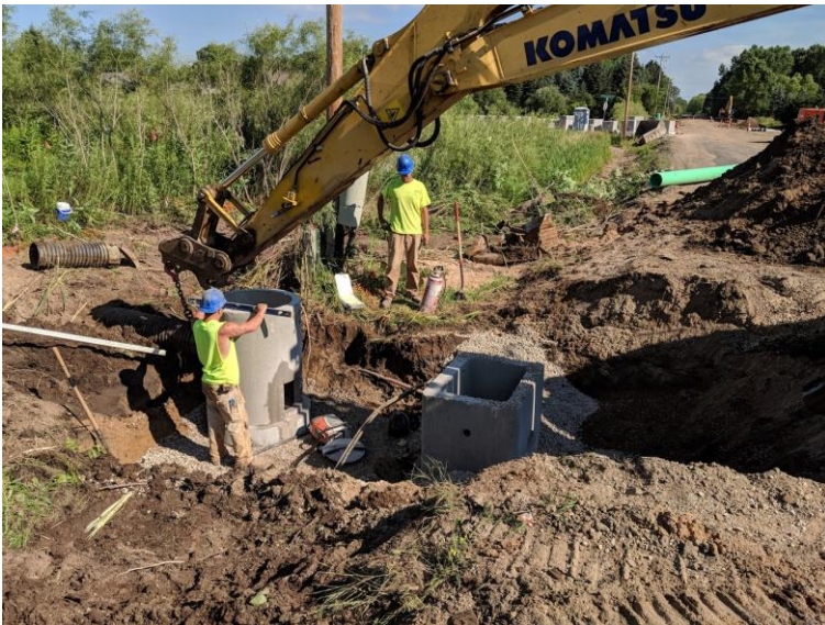
Setting Yard Drain For Retention Pond Outlet South of Starview Drive
