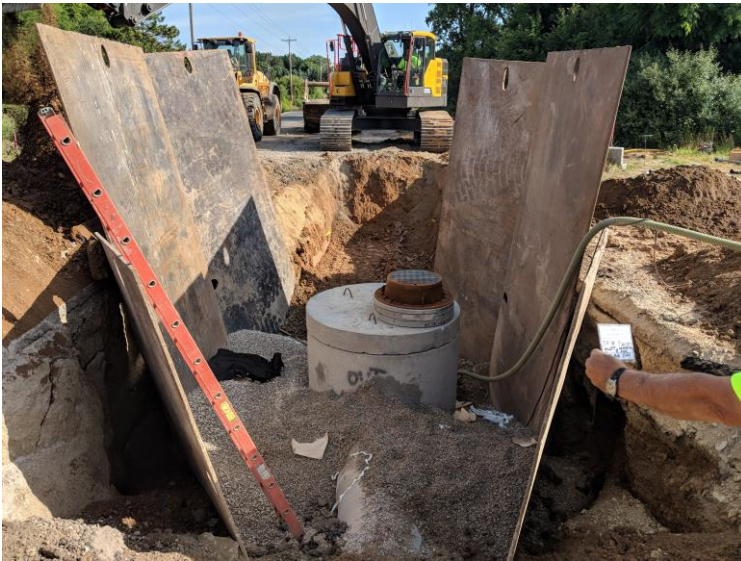
Setting Manhole at Skyway Lane
