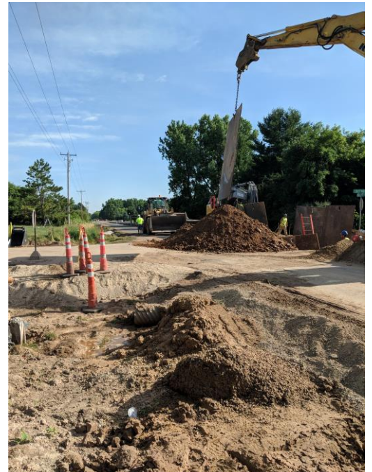
Installing Storm Sewer Main at Skyway Lane"
