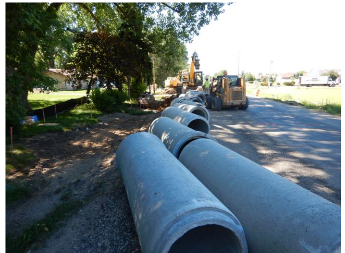
Storm Sewer Installation
