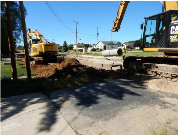
Storm Sewer Installation
