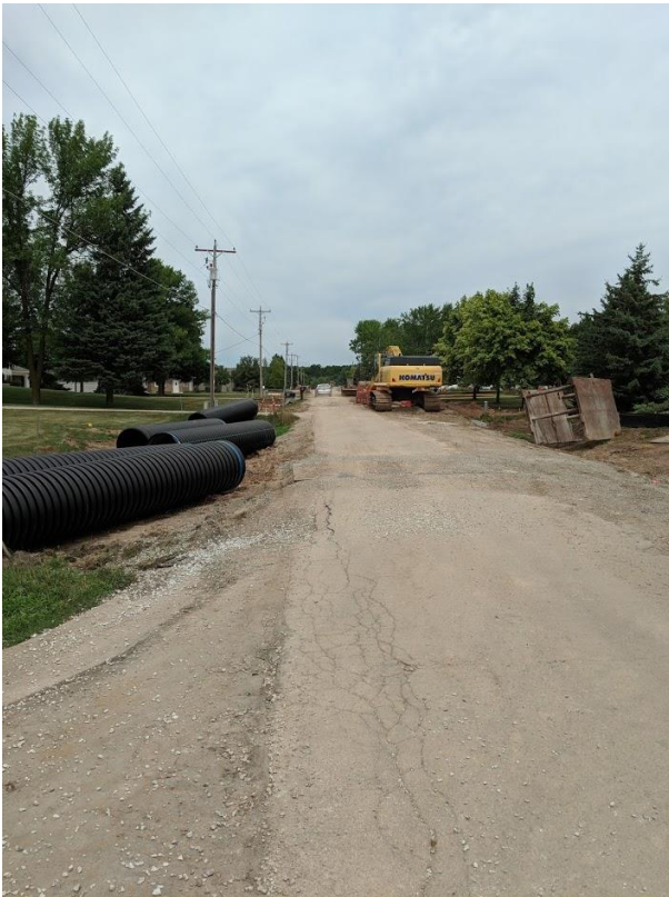
Installing Storm Sewer Main North of Amberwood Lane
