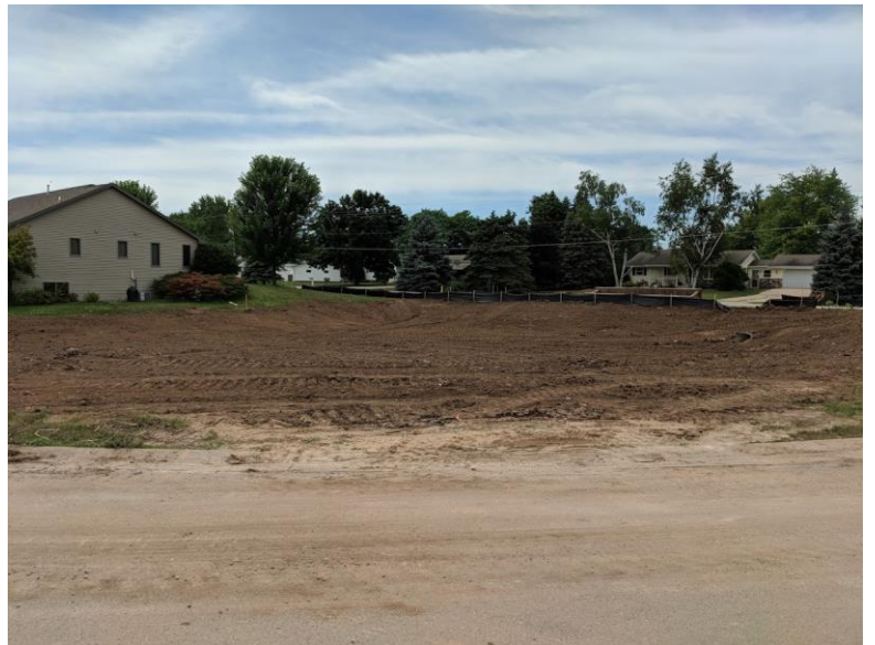
Rough Graded Detention Basin at Amberwood Lane and Casaloma Drive
