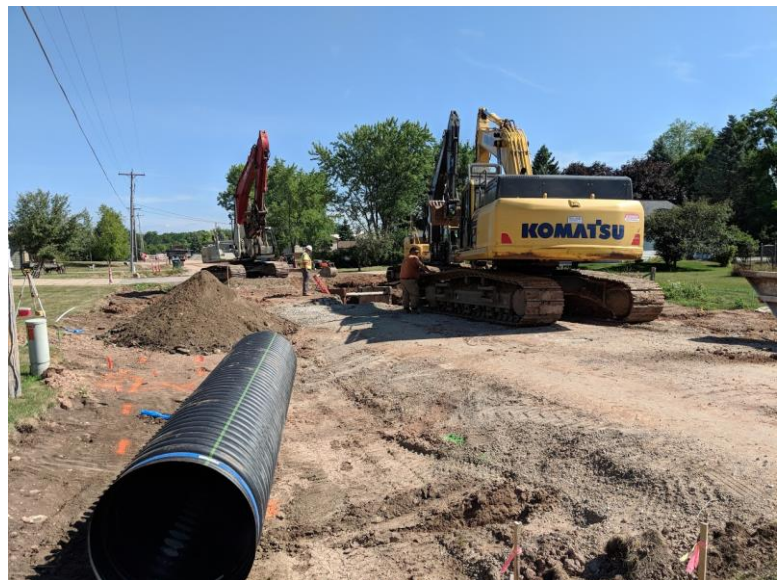
Storm Sewer Main Installation Operation
