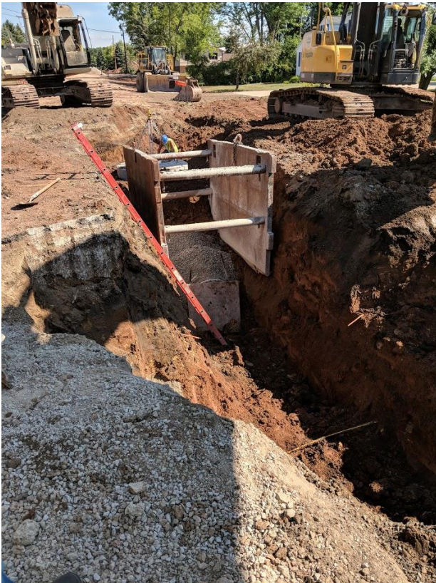
Installing Storm Sewer Main
