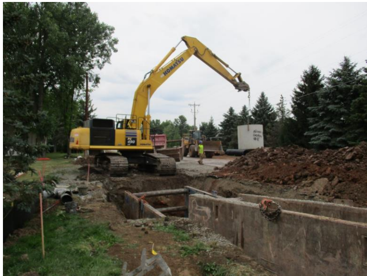
Installing Manhole at Prairie Song Lane
