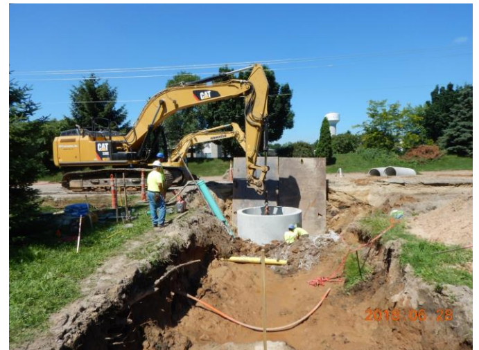
Setting Storm Manhole From Gillett Street to Retention Pond
