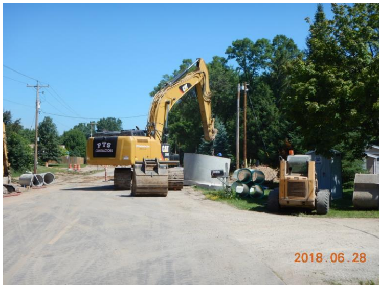
Storm Sewer Installation
