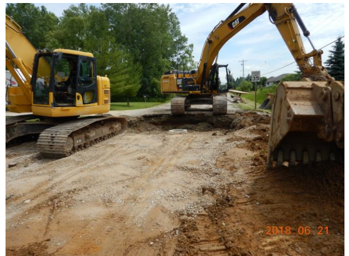
Sanitary Sewer Installation
