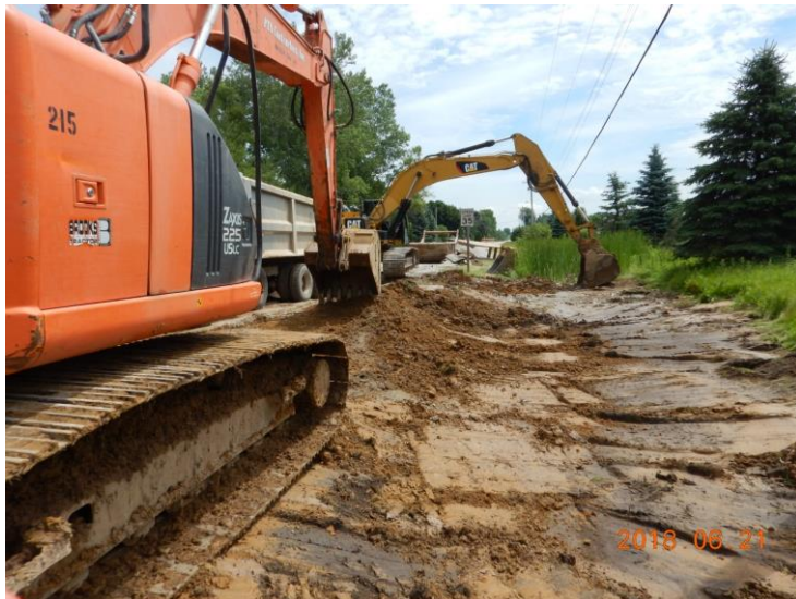
Stripping Topsoil
