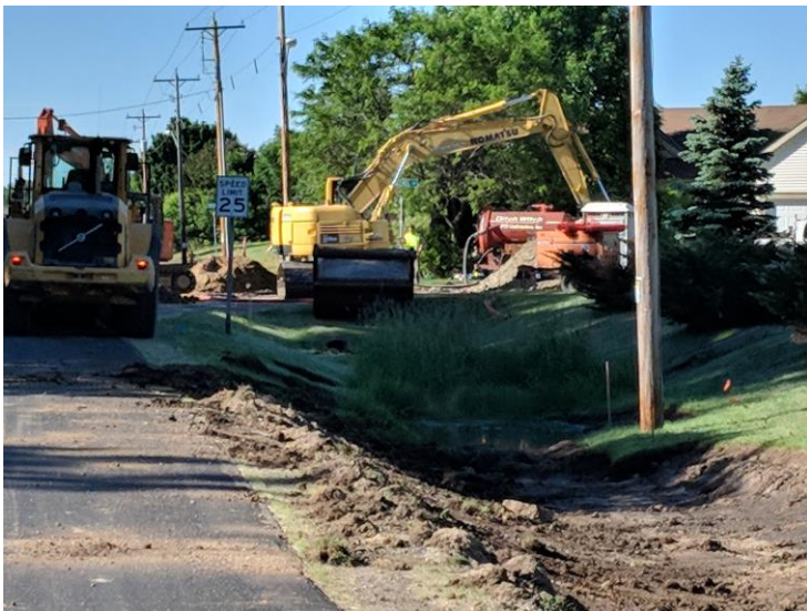
Water System Bolt Replacement
