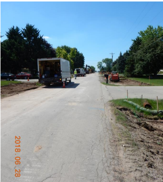
Utility Relocations & Bolt Replacements North of Capitol Dr
