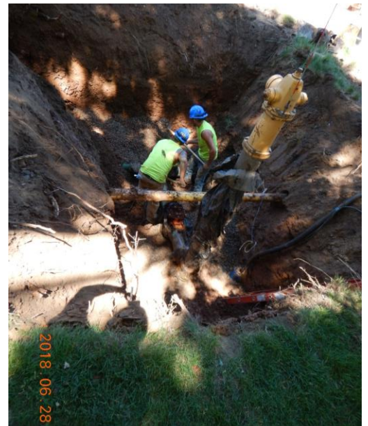
Water System Bolt Replacements
