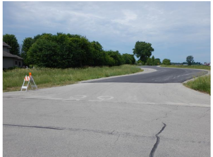
Temporary Access Road at Cobble Creek Drive
