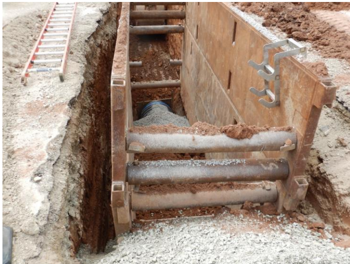
Storm Sewer Installation
