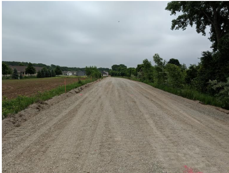
Temporary Access Road Grading
