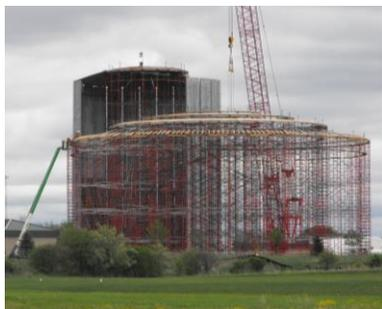
An 8.0 mg ground storage tank, 166' diameter, 50' tall will have 41 wall panels and 120 roof panels. There are no interior supports to hold up the tank roof. 332 miles of wire will wrap this tank. Tension on the wires will be 140,000 psi. This tank will provide backup water to the remaining four member communities. In addition, a booster pump station provides additional emergency supply to Ledgeview and Bellevue.
